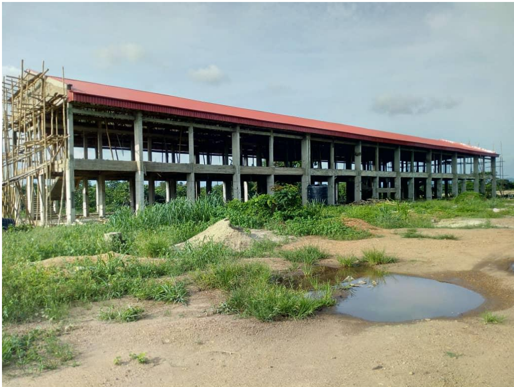
Figure 5.1: Nursing Department Building (Started in 2018) – [On-going at slow pace]
